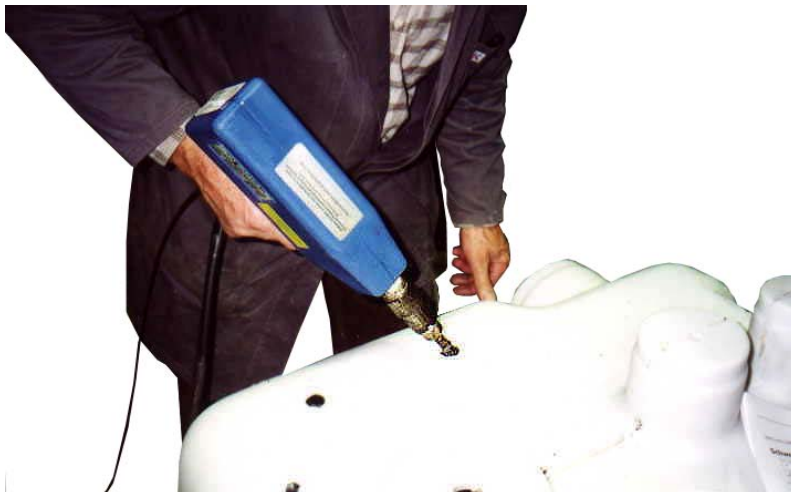
Fig. 1a: Repair of parts with the Drader Injectiweld (welded for the picture with black welding rod).
