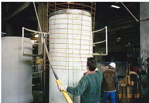
5. Bringing in the reinforcement.
