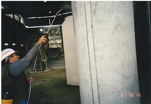
3. Moisten the anchor fleece material.
