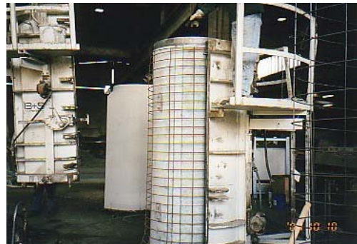
6. Latching of the formwork.
